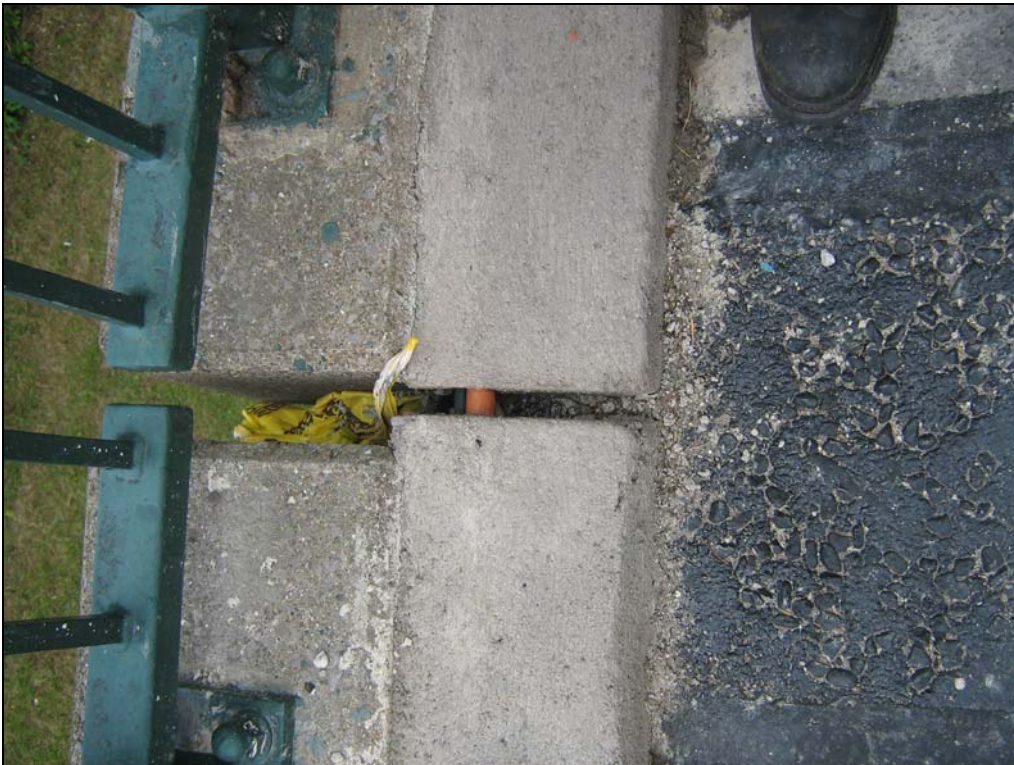
Photo 4: an example of services in the viaduct footway
