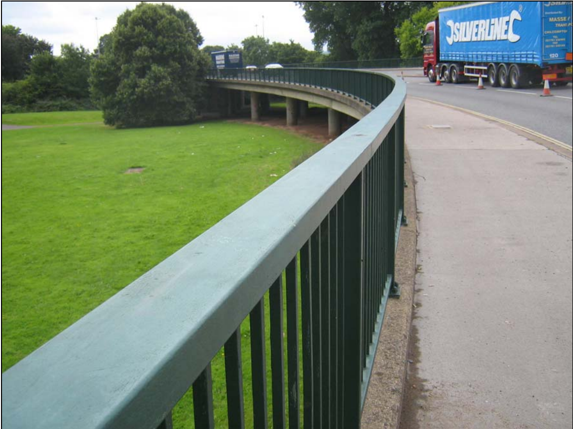
Photo 2: view along southbound parapet and footway
