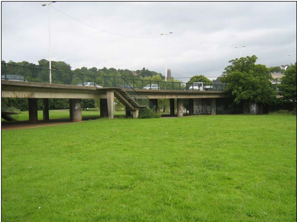
Photo 1: Brunel Way viaduct looking north east towards the Clifton Suspension Bridge
