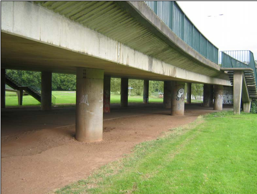
Photo 3: view along southbound viaduct cantilever
