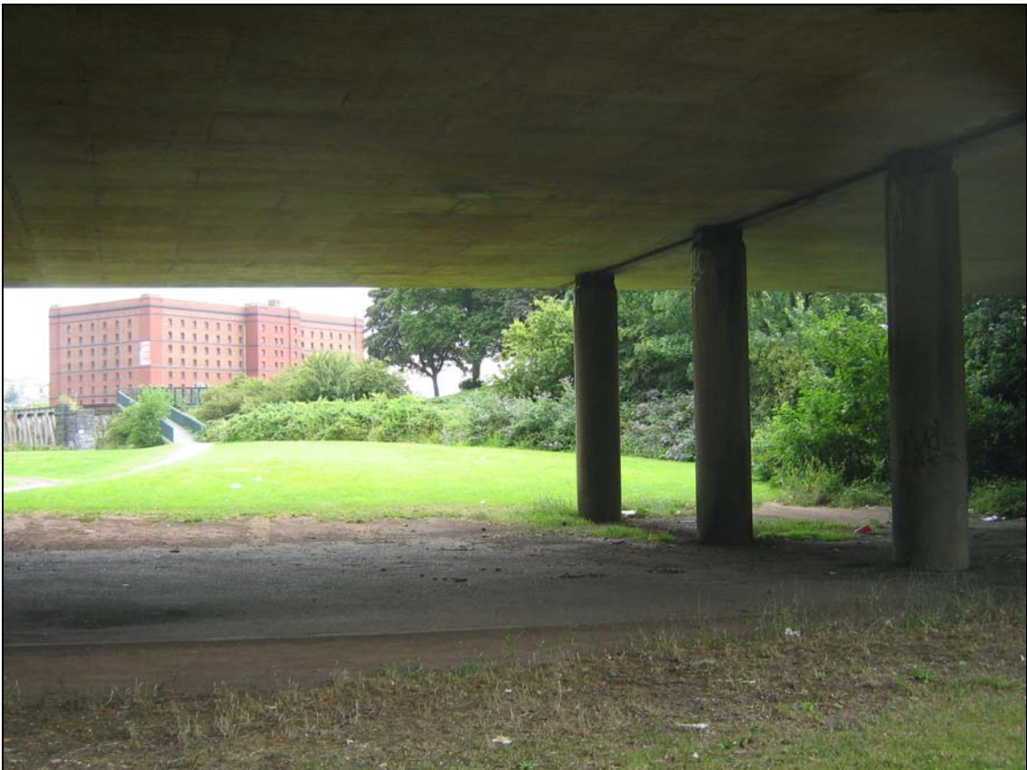
Photo 5: view under Brunel Way looking north east towards Ashton Avenue Bridge
