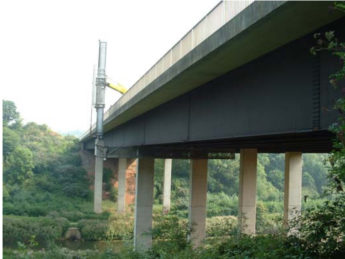
A4174 Ring Road Bridge Inspection (South Gloucestershire Council)
