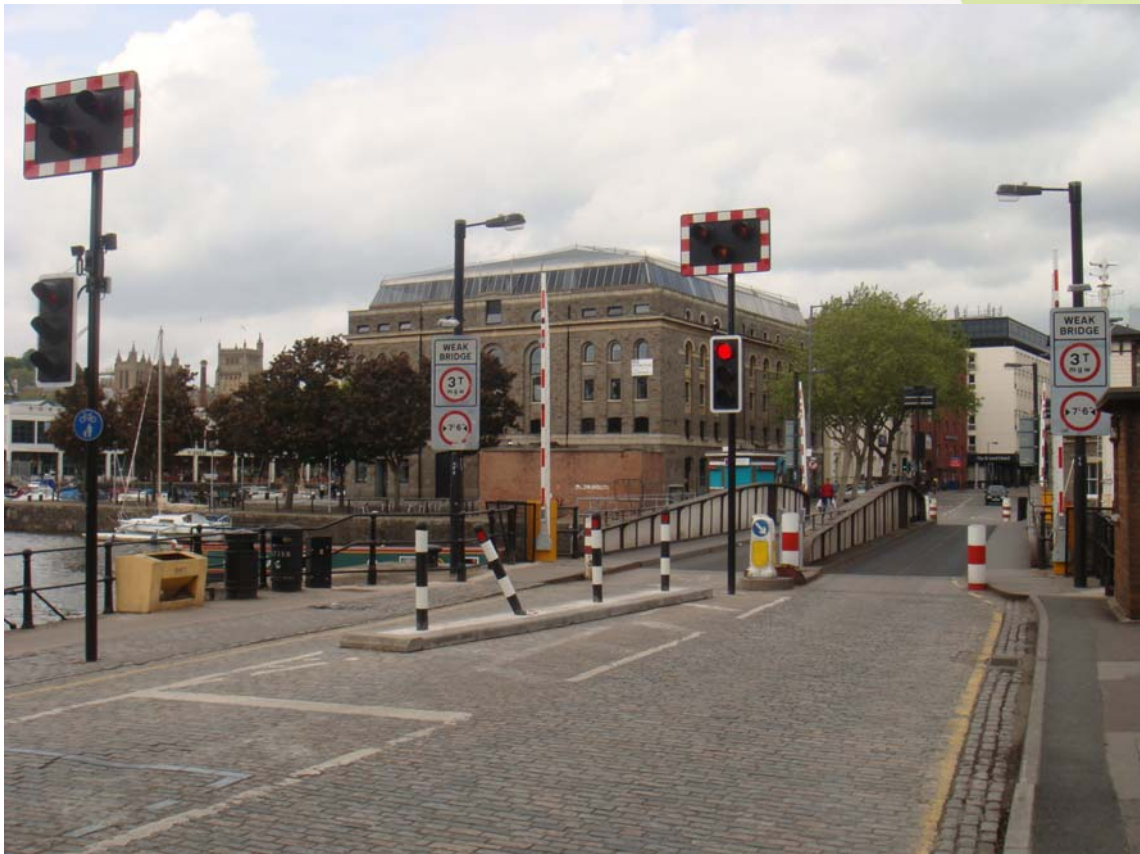
Figure 1 – Prince Street Bridge from South
