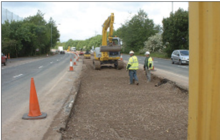
A4174 ring road 'Exceptional' maintenance scheme
